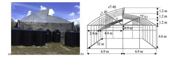
Figure I.9.1.1 Field trials of the Natural Ventilation Augmented Cooling (NVAC) greenhouse[15].
