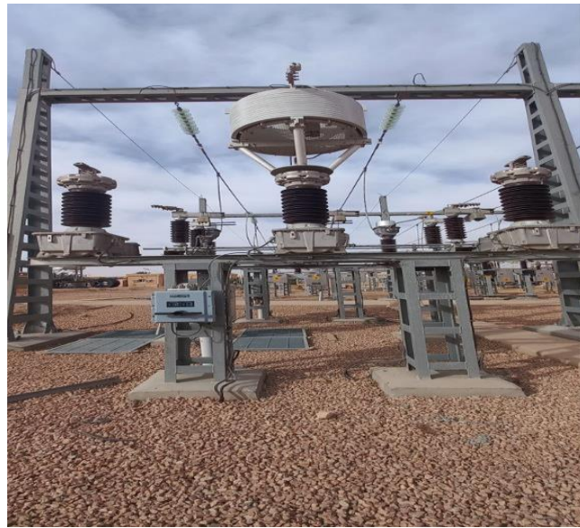
Figure II.12 : Photo de Circuit bouchon.
