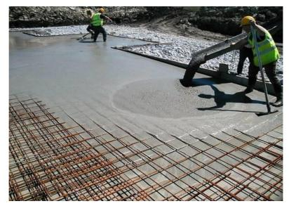
Figure (I. 1) self-compacting concrete
