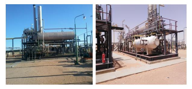
Figure IV.2. MEG regeneration unit(side A) Figure IV.3. MEG regeneration unit(side B)
