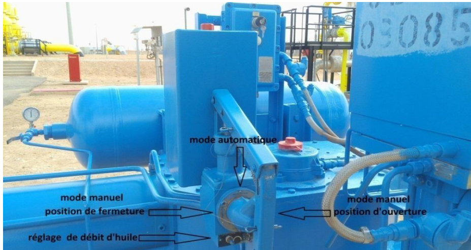
Figure. III. 3. Description de la pompe manuelle
