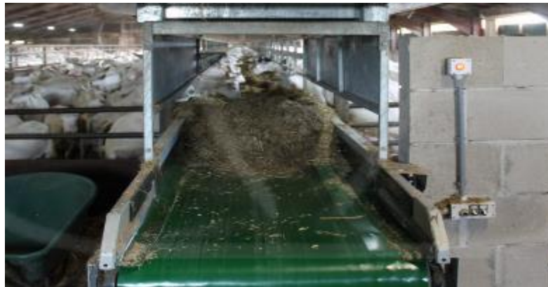
Figure 0-6 : Automatic feed distribution system by belt
