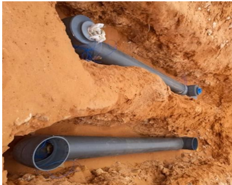
Figure III-5: Installation of the two tubes under the greenhouse floor.
