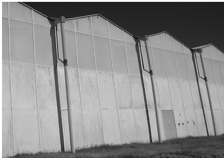
Figure II-19: Whitewash applied on the outside surface of the glazing [1].
