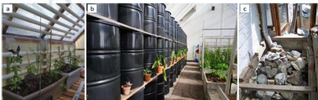
Figure II-2: Thermal heat storage mediums inside PSGs; a) PCM pipes (“Fashioning a Greenhouse: Hobby Greenhouse with PCM Pipes,” n.d.), b) Water barrels (“Tips on Using Water Barrels in a Solar Greenhouse | Cere Greenhouse,” n.d.), c) Rock bed (“Solar greenhouse - Ecodiy DIY eco-house,” n.d.). [30]
