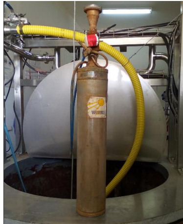
Figure 4.8 La pompe immergée (Water Max A64 DC).
