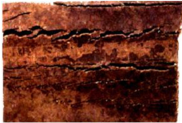
Figure I.10. Fissures de CSC [11]
