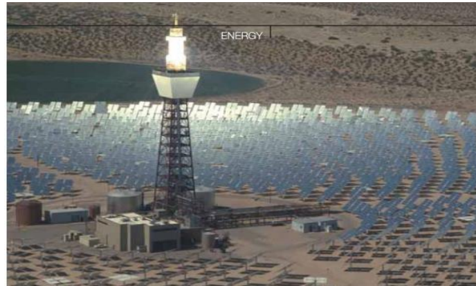
Figure.I.30: Solar II central receiver plant in Barstow, California [15].
