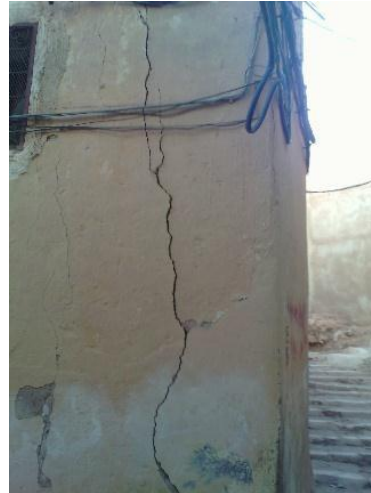
Figure 62: fissure verticale.
