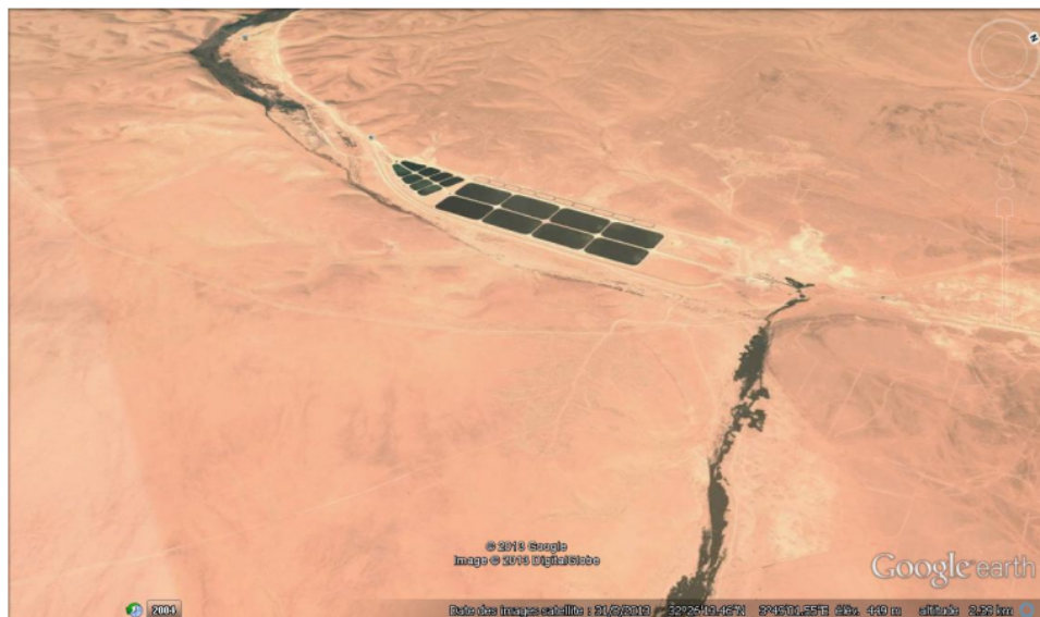
FIGURE 2.2 – Photo de la STEP (Google earth, 2013)
