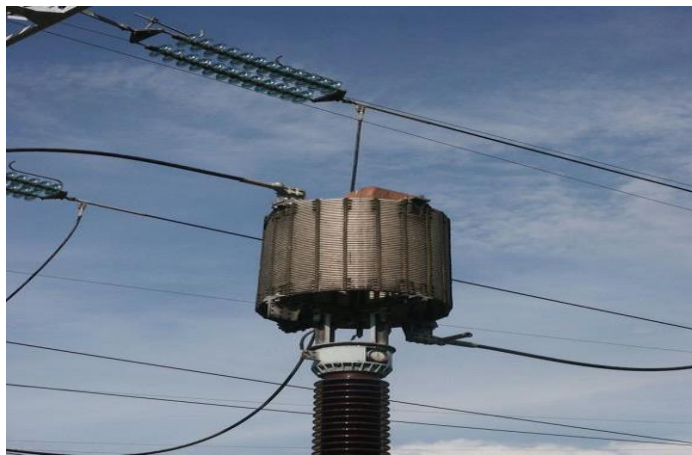
Figure II.10 : Circuit bouchon
