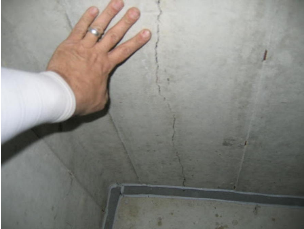
Figure 1.1: Crack detection by manual visual inspection (MVI).
