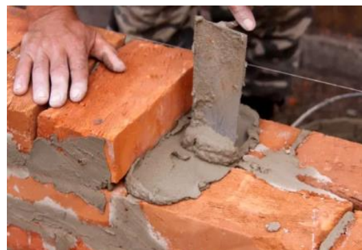
Master's Thesis – Civil Engineering (Structures) Figure 1.6: Laying of mortar for mortaring. Ref: [5].
