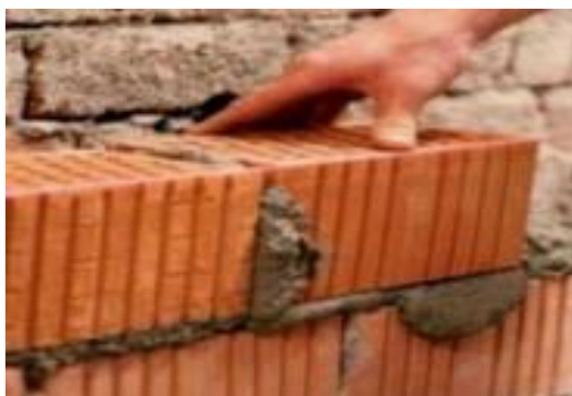
Master's Thesis – Civil Engineering (Structures) Figure 1.6: Laying of mortar for mortaring. Ref: [5].
