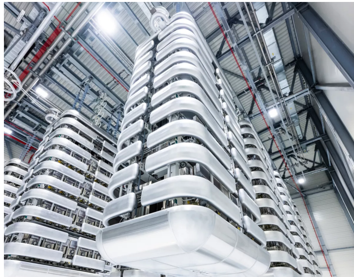
Figure 2.1: LCC valve hall with thyristor valves [40].
