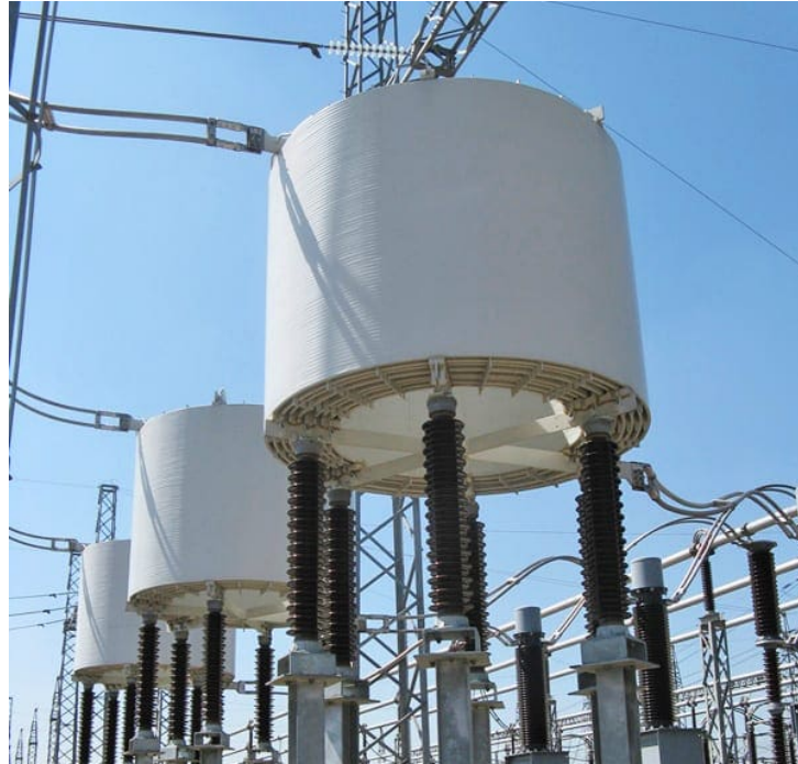
Figure 2.3: HVDC smoothing reactors [44].
