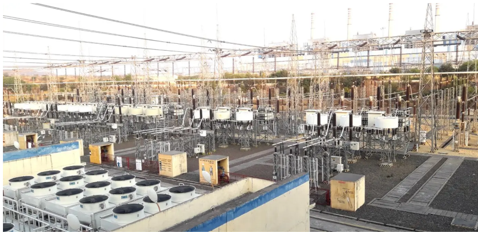
Figure 2.2: AC and DC filter reactors in an HVDC system [43].
