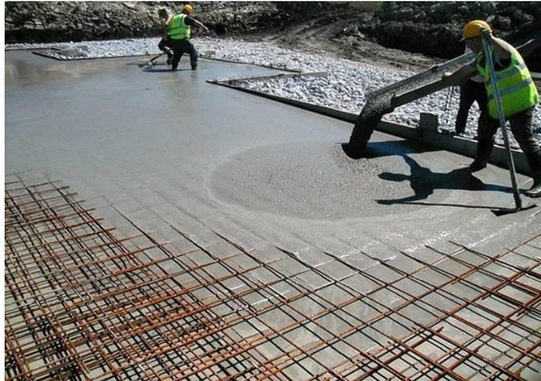
Figure (I. 1) self-compacting concrete
