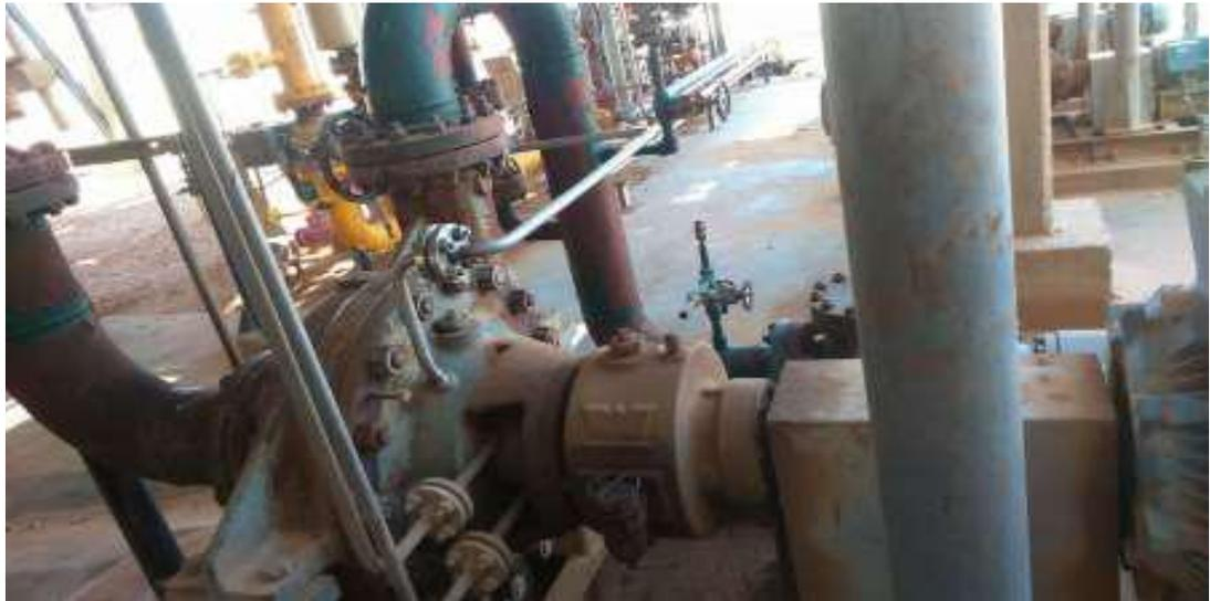
Figure V.13: Pompe transfère condensat 40-P-05 A
