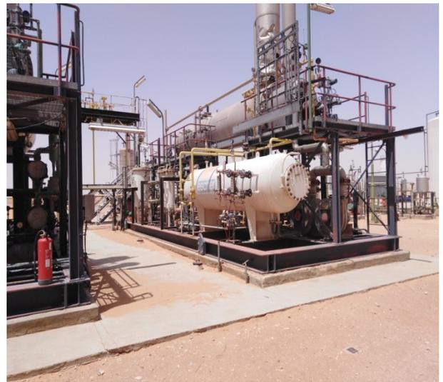
**Figure IV.2.** MEG regeneration unit(side A)      **Figure IV.3.** MEG regeneration unit(side B)
