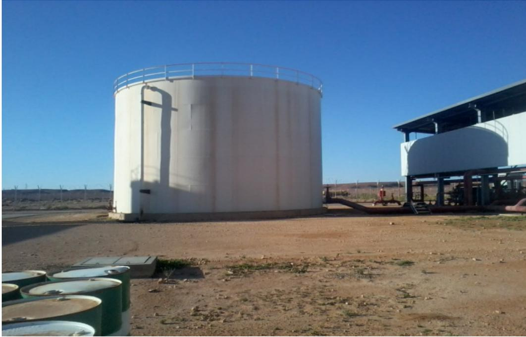
**Figure II.6.** water tank for Fire fighting
